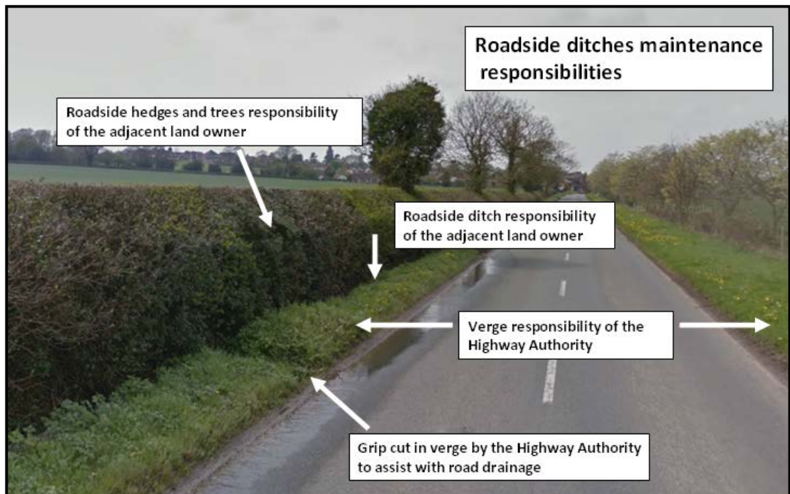
Figure 3-2: Responsibilities for Roadside Ditches and Watercourses
