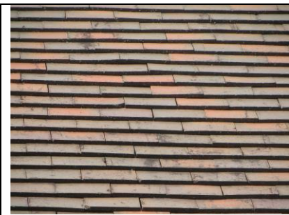
Showing gaps in roof covering.
