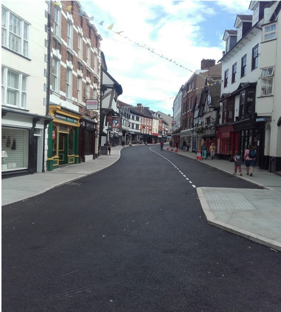
Mardol resurfaced and new paving
