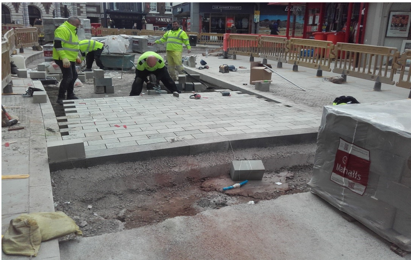
Laying york stone setts to carriageway from Mardol into Claremont Street
