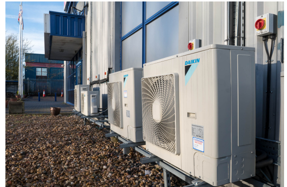
New energy efficiency units replaced old air conditioning
