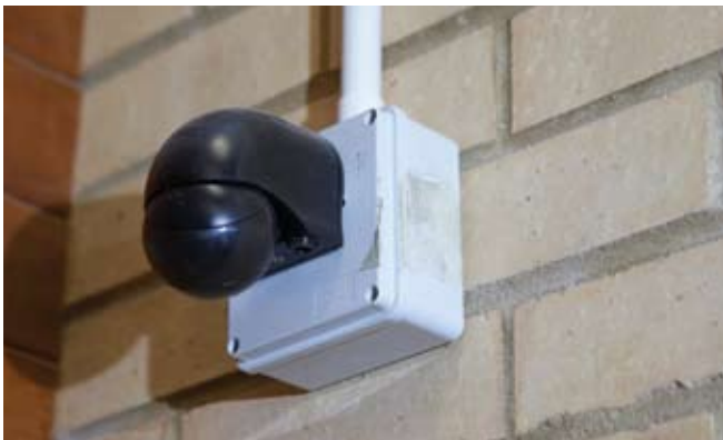
Figure 8 Occupancy control and daylight sensing technology can provide substantial savings
