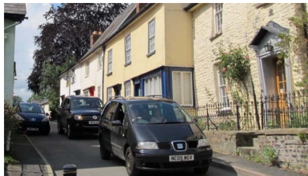
Welsh Street outside Moat House. Parked cars on left narrow the road
