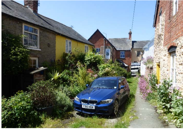
The shut accessed under the flying freehold at no. 26 High Street.
