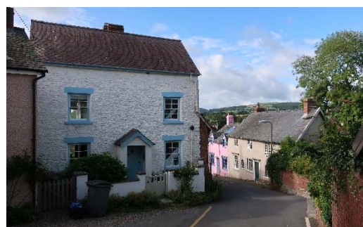
The view with Tudor House in the foreground
