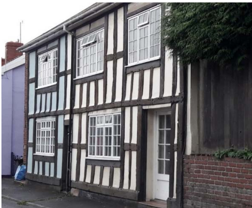
Half-timbered houses. Facades use traditional techniques
