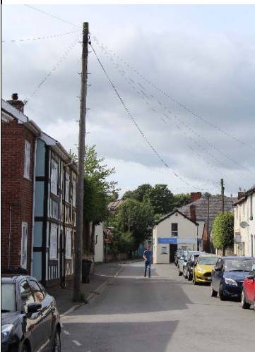
Intrusive overhead electricity cables
