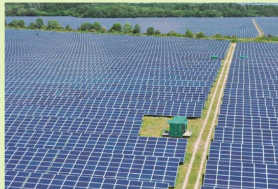
Ariel drone footage of a solar farm, W.Hitchcock, Above Surveying, Unknown
