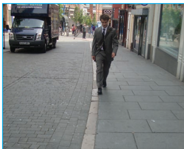
Kerb heights of between 75mm and zero (at informal crossings) were used with streetscape improvements in the centre of Nottingham.
