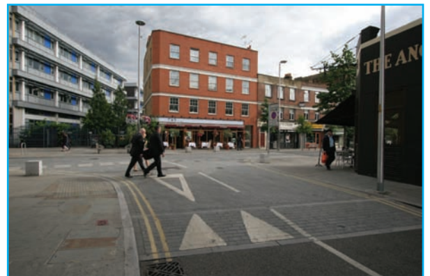
This junction has the Give Way marking (1003) and the approach triangle (1023) but no Give Way sign. It would have been possible to omit the approach triangle. Note also table to slow speeds and make pedestrian crossing easier.
