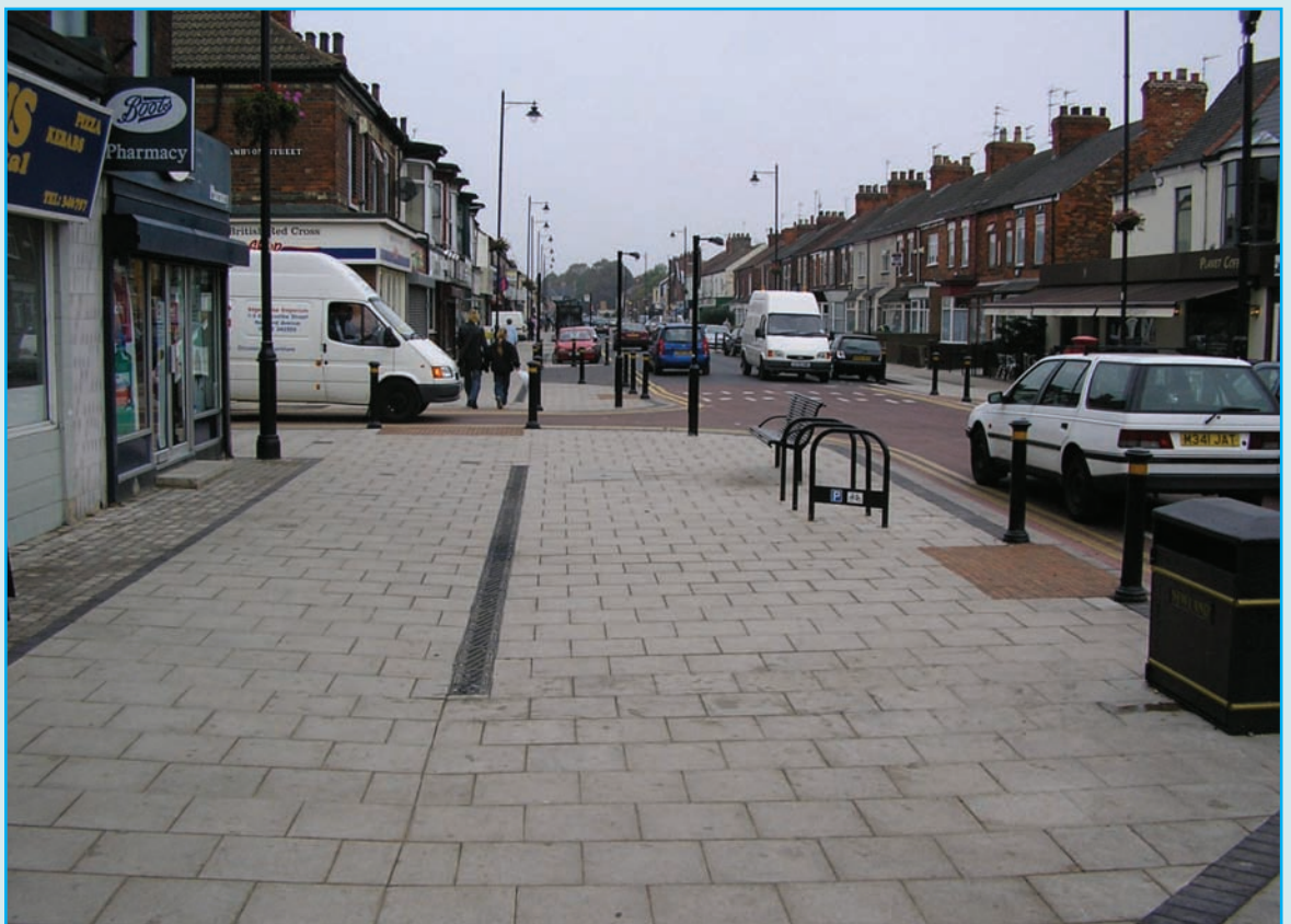
Footways widened significantly by narrowing carriageway
