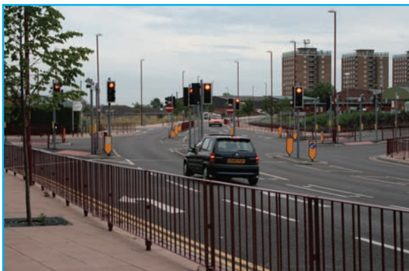
Newly-implemented highway scheme with extensive guardrailing
