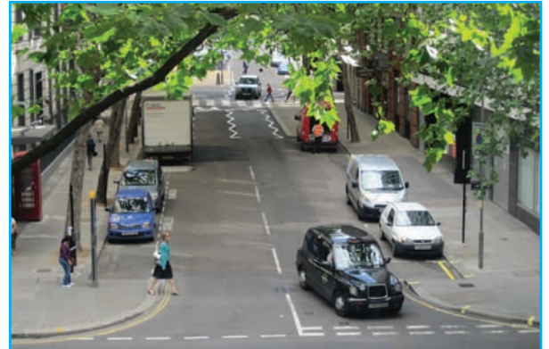
Well-integrated on-street parking.
