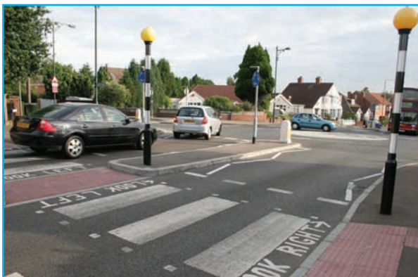
Zebra crossing close to mini-roundabout exit.
