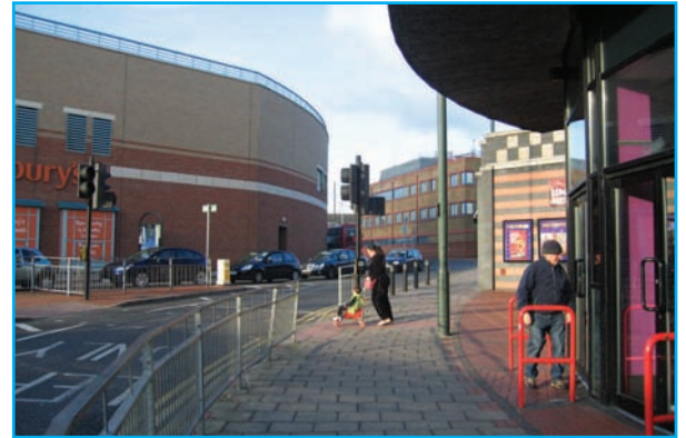
Segregated left turn lanes make pedestrian crossing movements more complex and slow, as well as adding to clutter.
