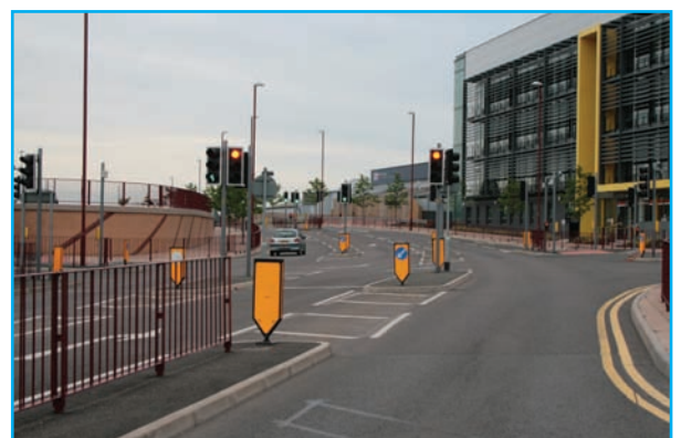
Multiple yellow retroreflective bollards can have a significant visual impact.
