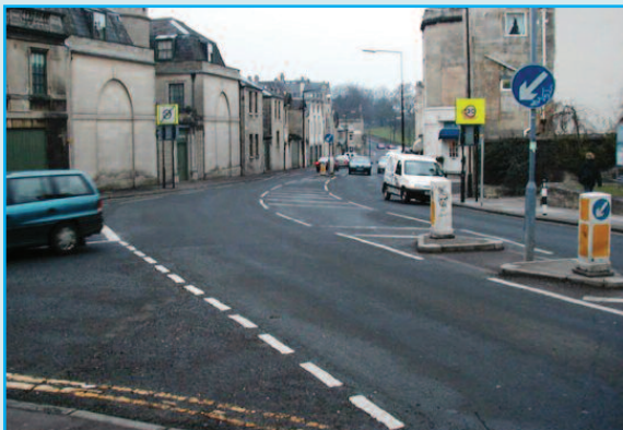
Julian Road Bath – Before and After
