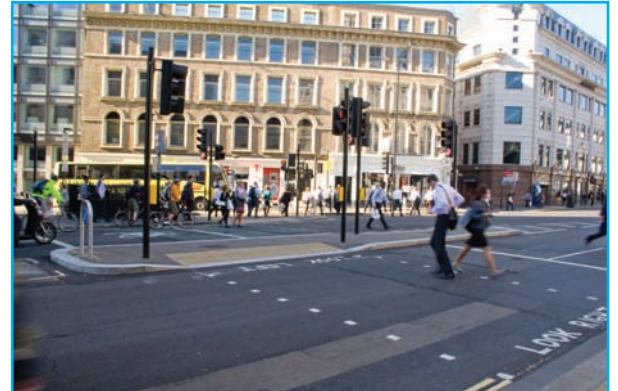
Staggered signalised crossing without guardrail
