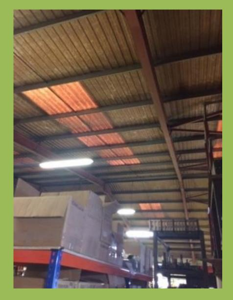
Example of very dirty sky lights and fluorescent lighting system, resulting in a very dark and poorly lit manufacturing space.
